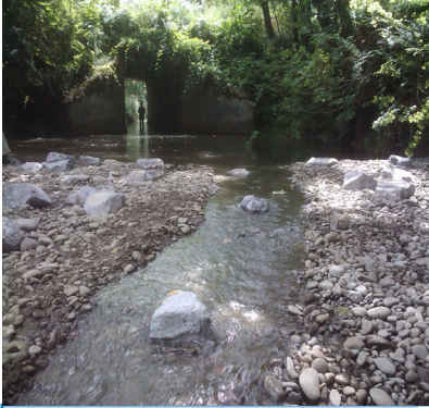
Completed Riffle at Redland Road
