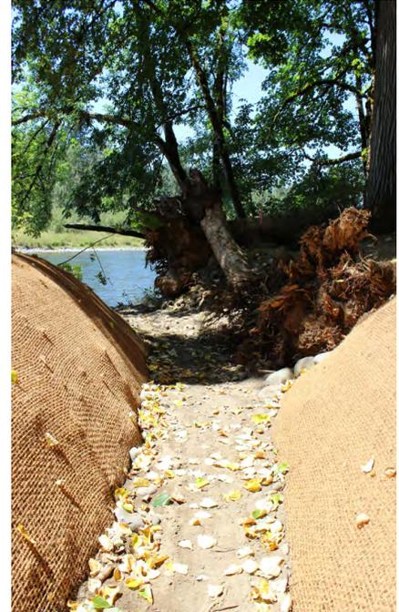
*Excavated side channel at Fishers Bend with erosion control mat*
