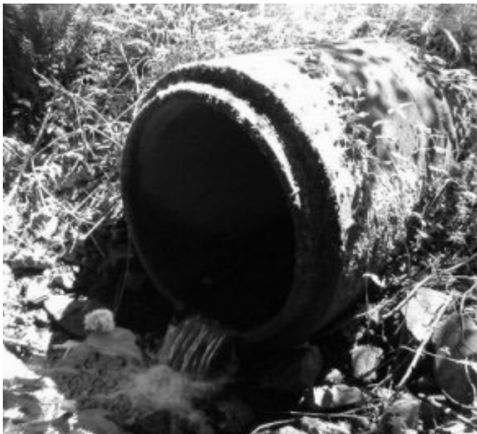
One of the 131 culverts assessed in the fish passage survey.
