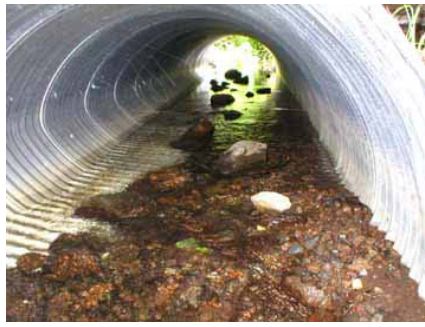
Notice the "natural" streambed in this culvert. Good for fish.
