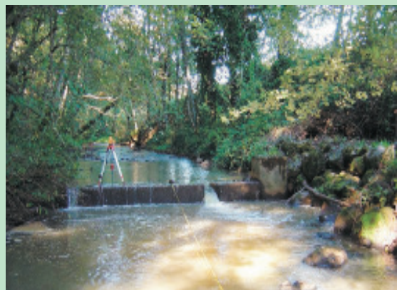
Fish can now travel through this area.
